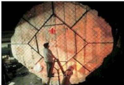
A 10-million BTU burner is being used for a refractory dry-out of a gas-fired pressure vessel
