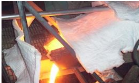
A 10-million BTU burner is being used for a refractory dry-out of a gas-fired pressure vessel
