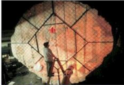
A 10-million BTU burner is being used for a refractory dry-out of a gas-fired pressure vessel
